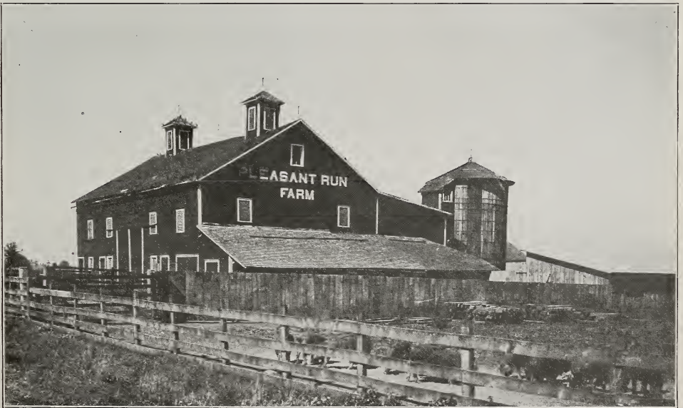
Where the Matrons Are Housed in Winter
